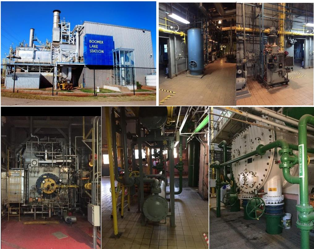
The dominant feature of the development parcel is the Power Generation Building. The skin of this building is stainless steel. The interior is filled with vintage power generation equipment still in operational condition. The building underwent various renovations during the 1990's. Most of the asbestos was removed during these renovations (the Unit 2 boiler has the only remaining asbestos and it is encased). No tests have found the presence lead-based paint.
